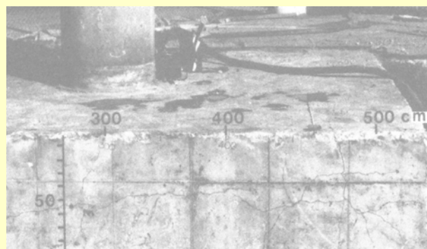
Cracks of field concrete caused by the Alkali Silica Reaction (ASR)
